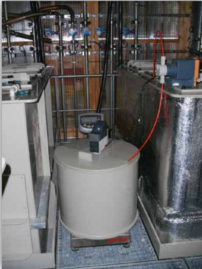
Addition of silver using pump
